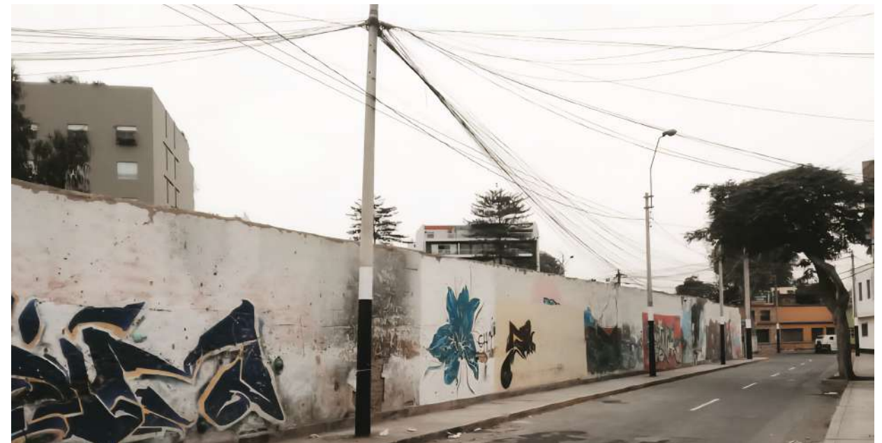
Existing buildings issues
